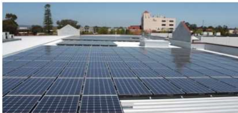
Figure 1: Rooftop PV System in Australia [2]
